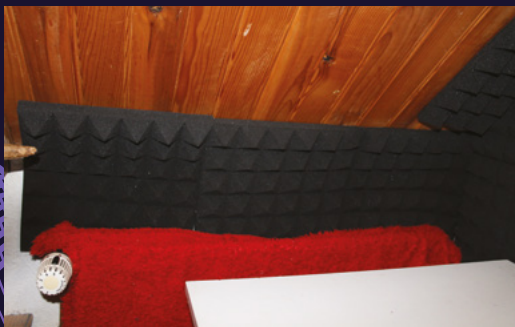
▲ Radiators can produce ringing echoes. Because we also like being warm, we covered ours with a fleece blanket for easy removal.
